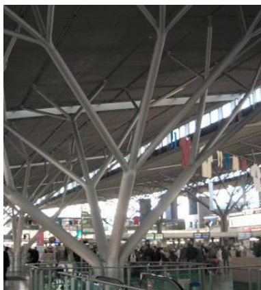
Fig. 4: Tree supports of Stuttgart Airport Terminal
