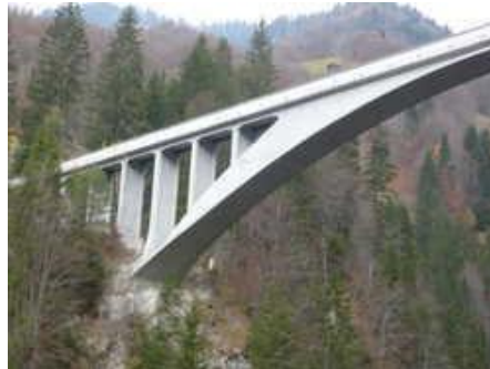
Fig. 6: Salginatobel Bridge – changable cross section.
