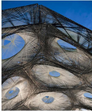
Fig. 5: Glass and carbon fibers structure of research pavilion ICD/ITKE, Stuttgart.
