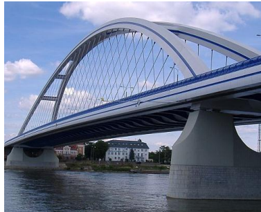
Fig. 2: Parabolic shape of bridge in Bratislava.
