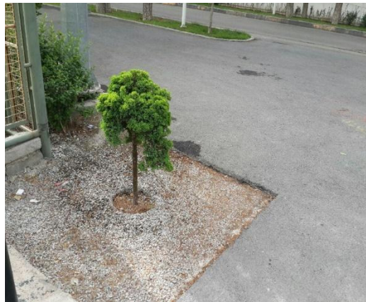
Fig. 1: pervious concrete pavement slab
