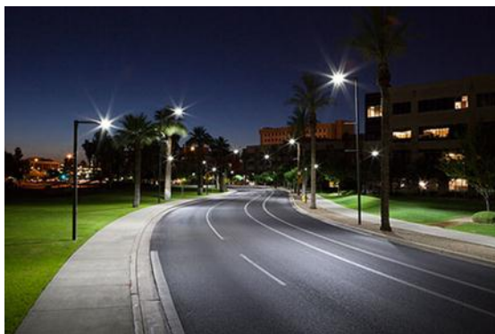
Fig. 1 A road being lit by LED Luminaire
