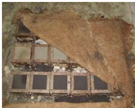
Fig. 4: Aerated concrete covered with gunny sack
