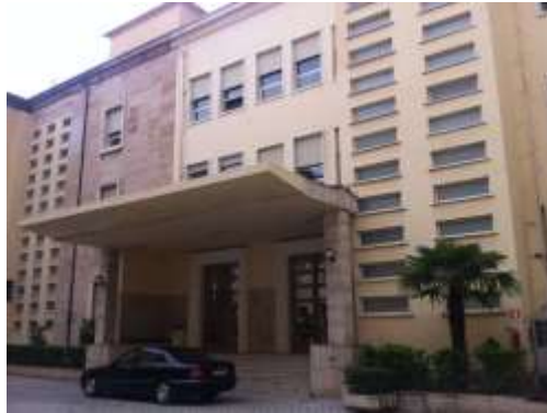
Fig. 1: View of the structure
